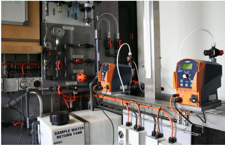
Figure 6 – Dosing pumps of TDU
