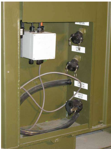
Figure 1 - TDU© services connection box
