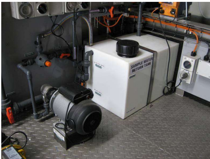
Figure 5 – Sample Water Return System, comprising sample water storage tank and return pump.
