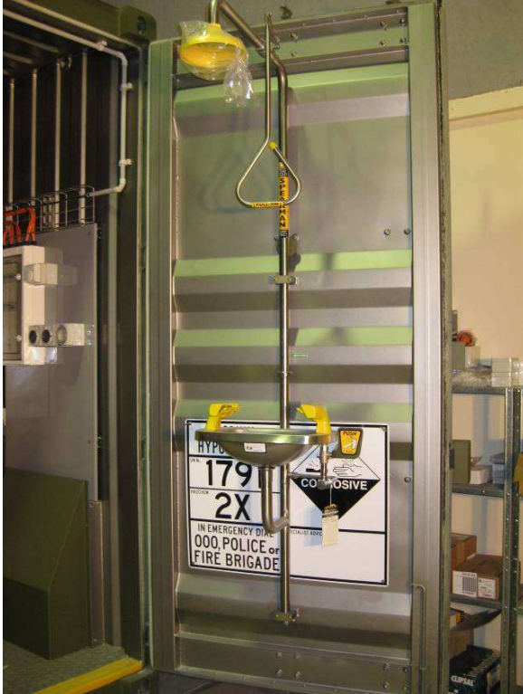
Figure 8 - Emergency Shower/ Eyewash installation shown in transport storage location
