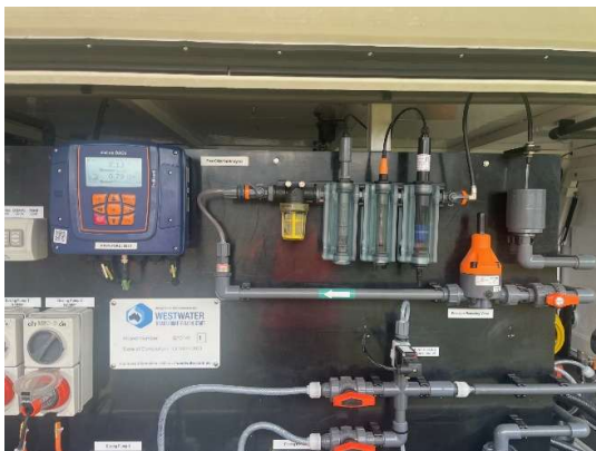
Figure 4 – PDU Typical Analyser Systems Arrangement,
