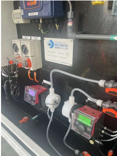
Figure 6 – Typical dosing pump arrangement for PDU
