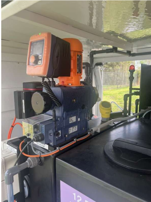
Figure 5 – Sample Water Return System, comprising sample water storage tank and return pump.
